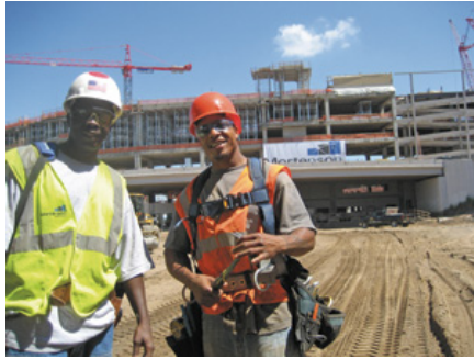
Eddie Jackson and Artie Crawford worked on construction of the new Target Field stadium as a part of Summit Academy's 100 Hard Hats program, a community-based, skills-focused training effort that combines community services, vocational training and employer services. - Photo: Elliot Stewart-Franzen
